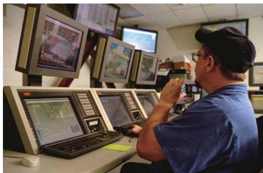
Figure 3: Wide Area Monitoring Systems (WAMS) and other advanced Network Management functions enable grid operators to proactively detect grid disturbances.
