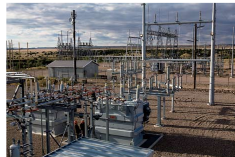
Figure 2: A new modular substation, built by ABB in Colorado for a major U.S. utility. Substation automation using IEC 61850 standards will help utilities better monitor equipment on the new smart grid.
