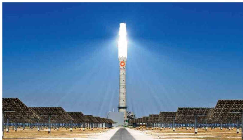
Figure 2: Molten nitrate salts flow through the 140-meter-high tower where they are heated to 565°C.
