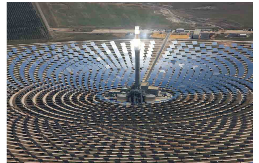
Figure 1: The facility's 2,650 mirrors reflect the sun's rays towards the top of the tower
