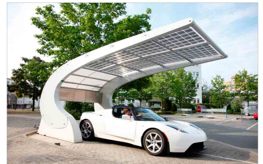
Figure 1: The solar carport from Evonik Industries takes advantage of the Evonik Plexiglas's transmission properties, which align well with the spectral response of solar cells.
