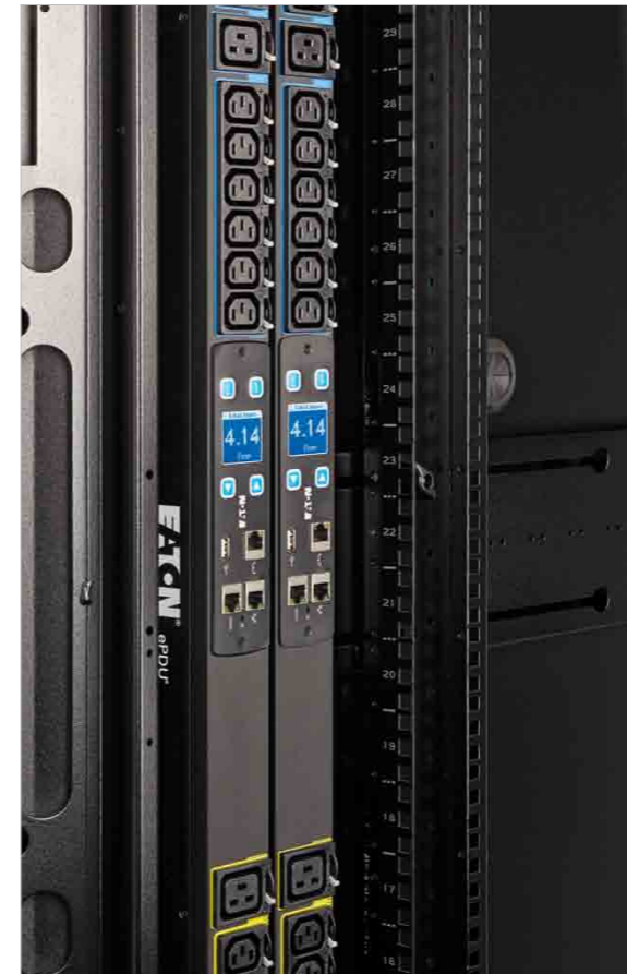
Figure 2: Rack capacity is used to select the appropriate input plug for the rack PDU
