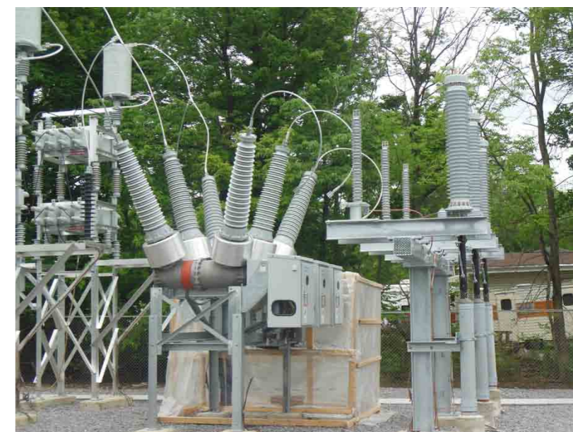
Figure 1: Big Tree Substation
