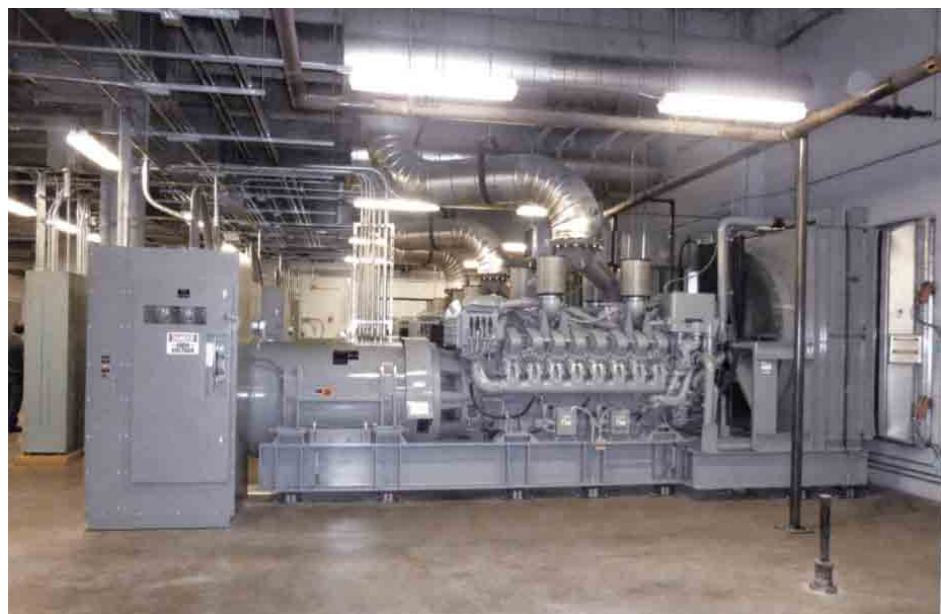
Figure 2: The MTU Onsite Energy generator sets meet EPA Tier 2 emissions requirements
