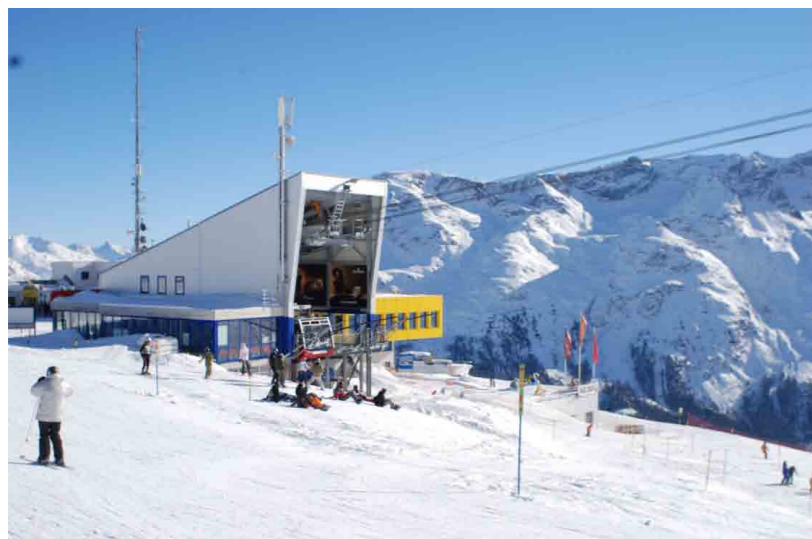
Figure 2: The complex network architecture of the entire ski resort using optic fiber
