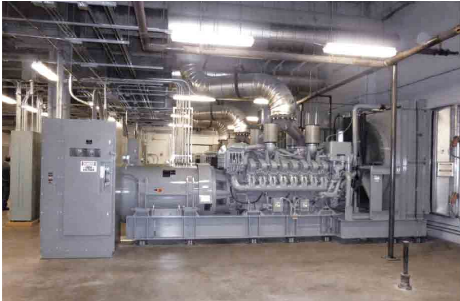
Figure 2: The MTU Onsite Energy generator sets meet EPA Tier 2 emissions requirements
