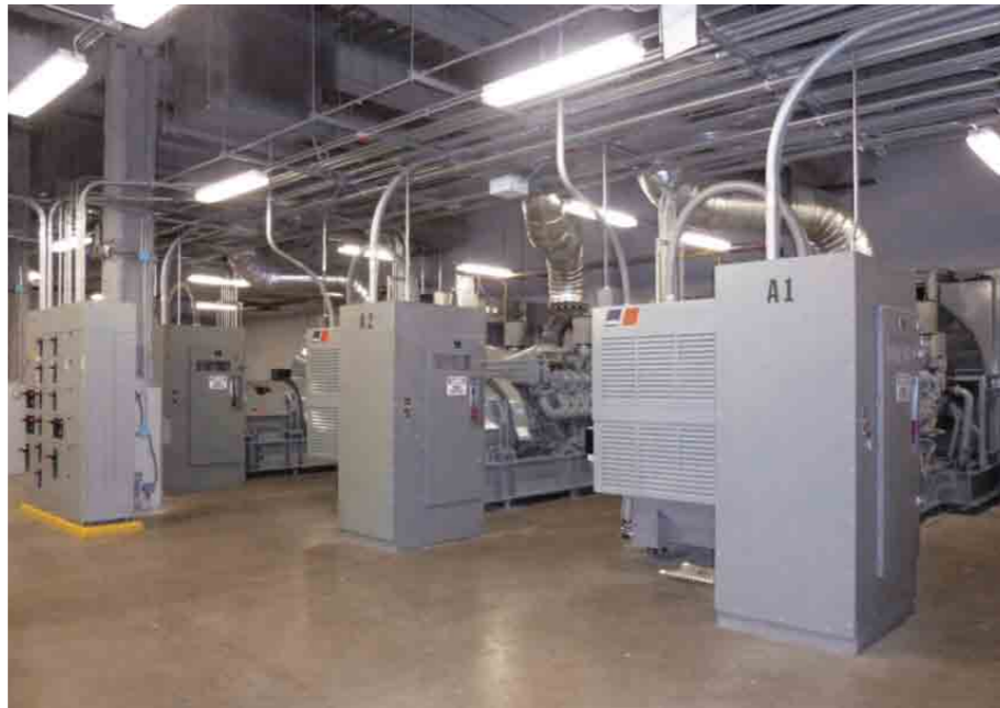
Figure 3: The medical center's emergency power system includes six 2,000 kW generator sets from MTU Onsite Energy
