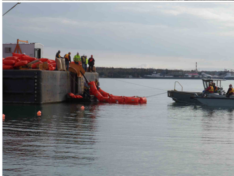
Figure 3: Engineering made the decision to pull the cable from the Drummond side to the DeTour side
