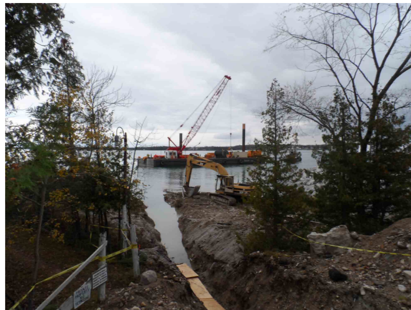
Figure 1: Kerite used a subcontractor to dig trenches and install the cable
