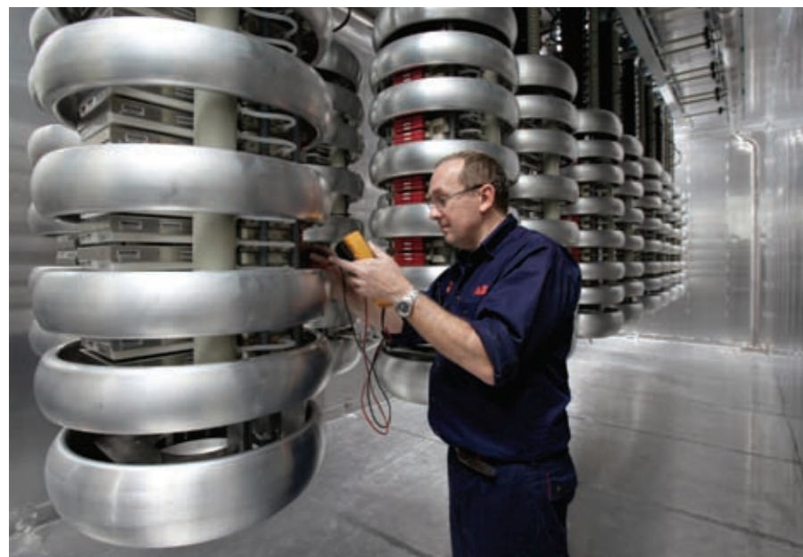
An ABB engineer tests HVDC Light valves to be used for the connection of a remote offshore wind farm north of Germany in the North Sea.
