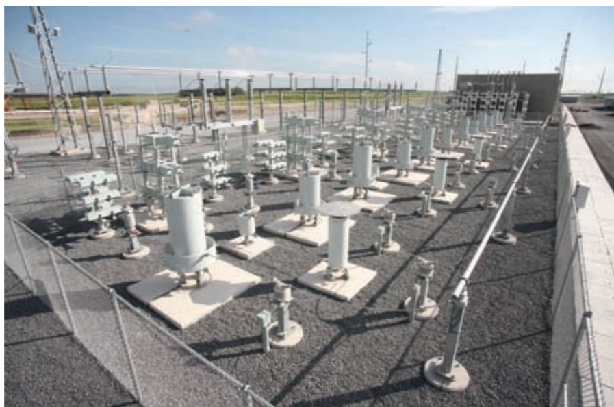
High-voltage direct current (HVDC) systems, like this Sharyland HVDC station connecting power grids between Texas and Mexico, enable bulk transmission across long distances.
