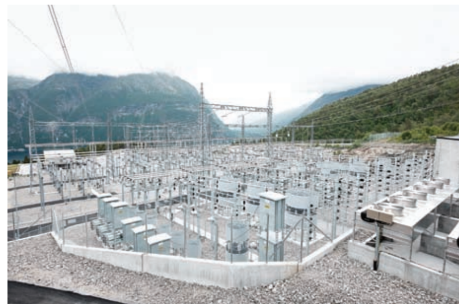
Flexible AC transmission systems (FACTS) enable and support remote variable generation with great reliability.
