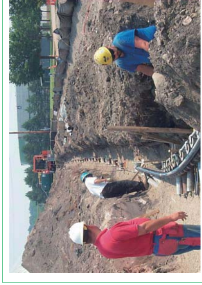
Figure 4: HVDC Light cable laying with minimum environmental intrusion.
