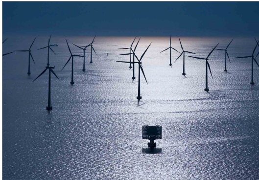
Figure 1: Offshore wind park “Lillgrund” in Sweden is connected to the main land via a 138kV high-voltage DC link
