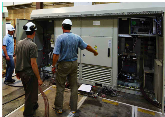
Figure 2: Performance evaluations at independent test facilities, such as DNV KEMA's FPGL (Flex Power Grid Laboratory), can assure both supplier and operator that inverters perform to utility requirements.
